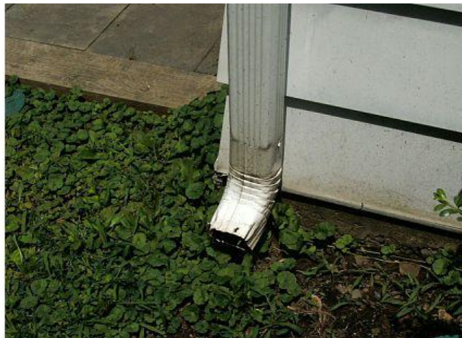
Downspout at base of home
