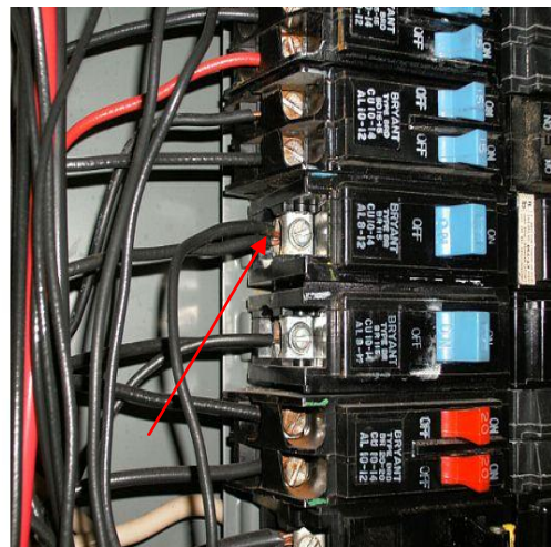
Double tapped circuit breaker
