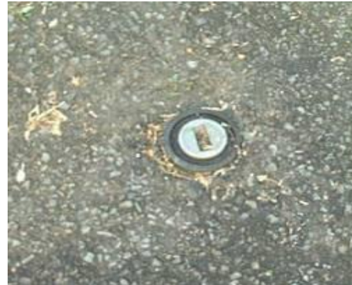
Old oil lines and an oil fill in the driveway indicate presence of an abandoned buried oil tank
