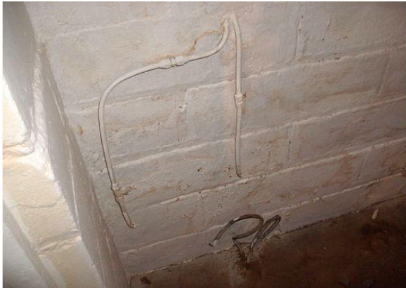
Old oil lines and an oil fill in the driveway indicate presence of an abandoned buried oil tank
