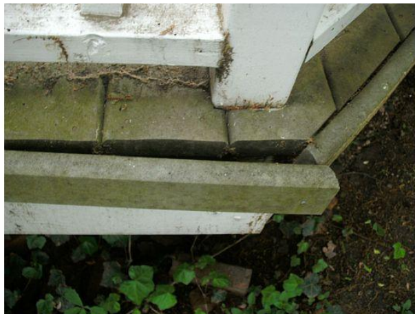
Detaching perimeter board
