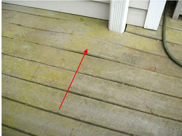
Tightly set and warped composition deck boards
