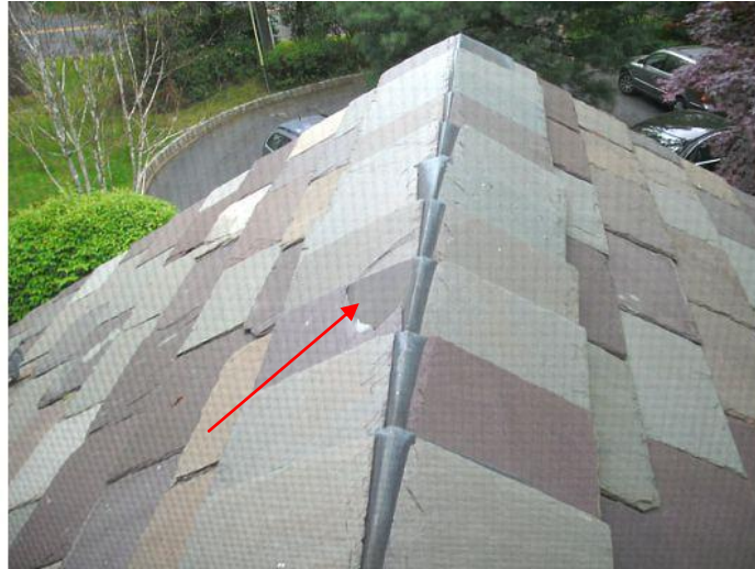
Cracked roofing
