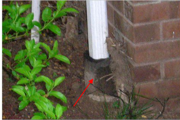
Older tarpaper underground pipe
