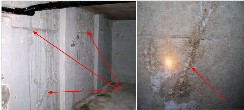
Water Entry & Damage to the Masonry Foundation at Front and also Crack and Water Entry thru Ceiling
