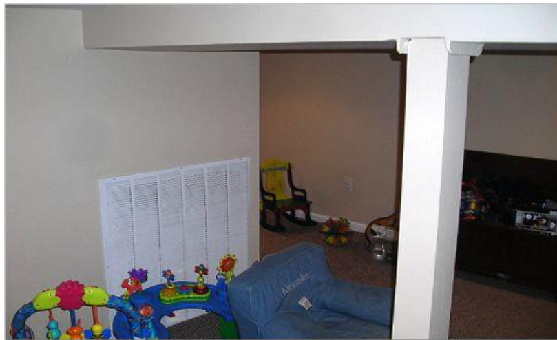
Basement is newly finished with fixed walls everywhere, and no access to utilities'
