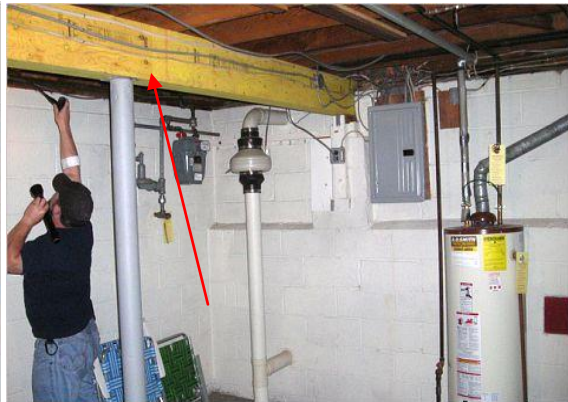
New beam installed, near left front
