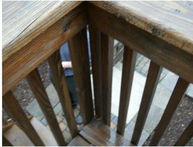
Doubled balusters instead of corner railing posts
