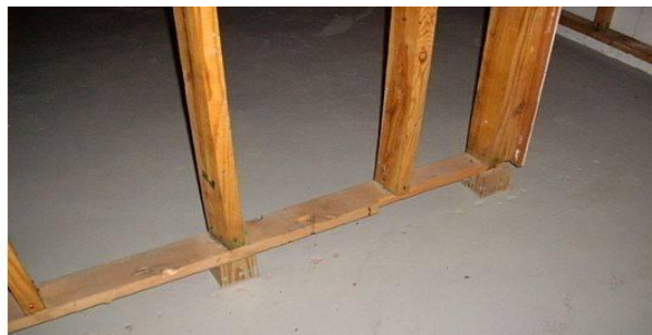
Wood stud wall is raised off basement floor by blocks
